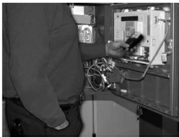
Figure 3.2 — Keep one hand in a pocket or behind your back when testing energized equipment to avoid creating a path for shock current.
