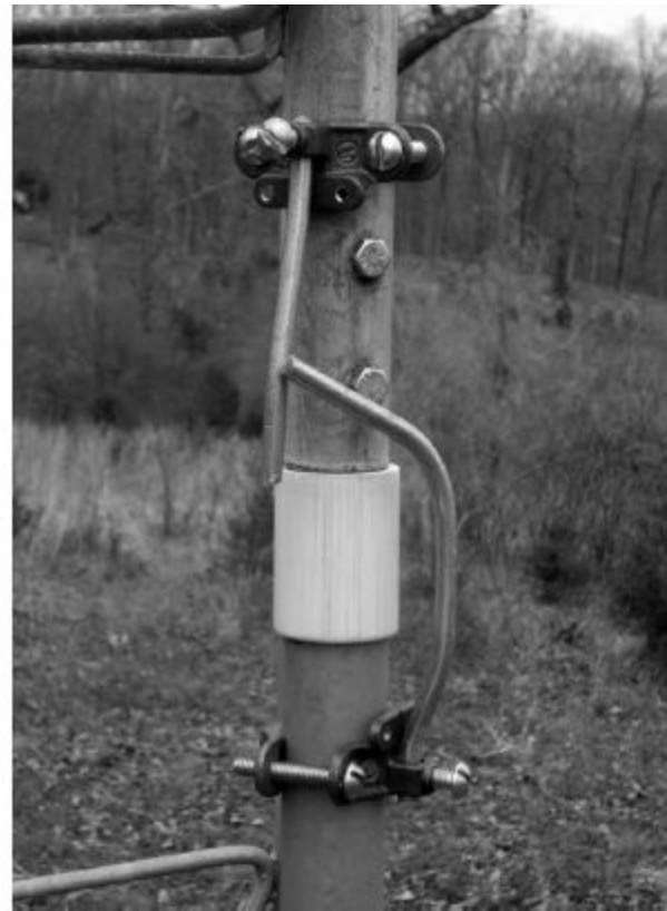
Figure 4.12 — Pipe spark gap constructed by Tom Rauch, W8JI (A) and a wire-and-clamp spark gap constructed by the author (B). [Photo for 4.12A courtesy Tom Rauch, W8JI]
